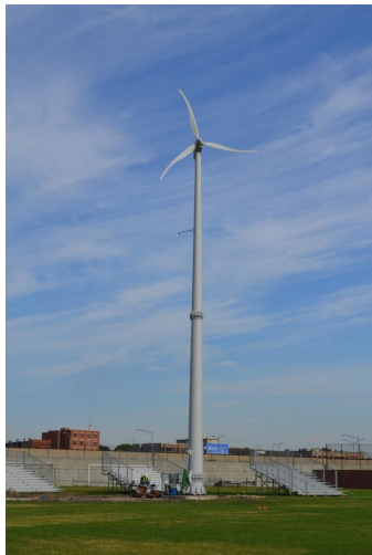
Turbine on Tower: 7/14
